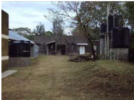
Fig 21 – Partially complete Main Hall
