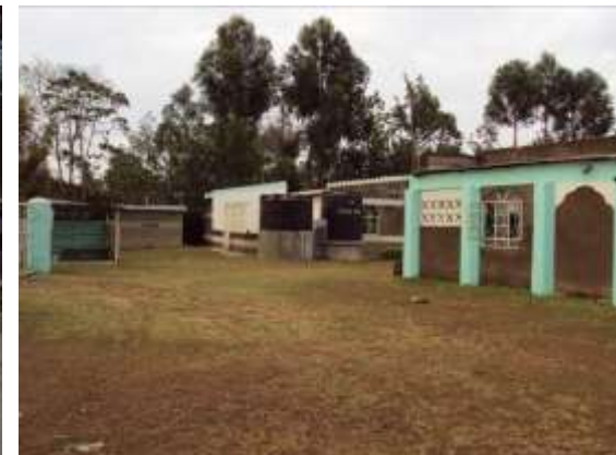
Fig 23 – Water Storage Tanks
